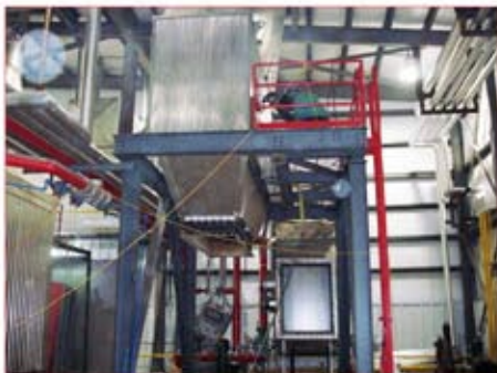
New Installed Economizer
